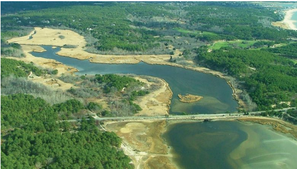
Restoring the estuary's tidal flows hinge on replacing the 1908 dike with a new bridge and two secondary dikes. With strong partnerships and funding, we hope to start construction in 2018. © Friends of Herring River.
