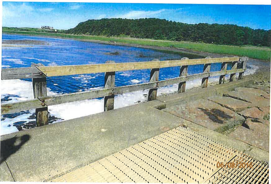
Photo 14: Rail at west has been repaired.
