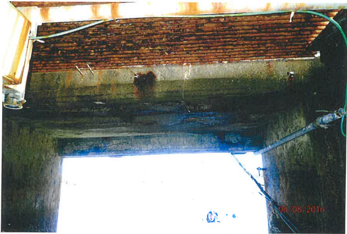
Photo 1: Roof of south upstream flume extension.
