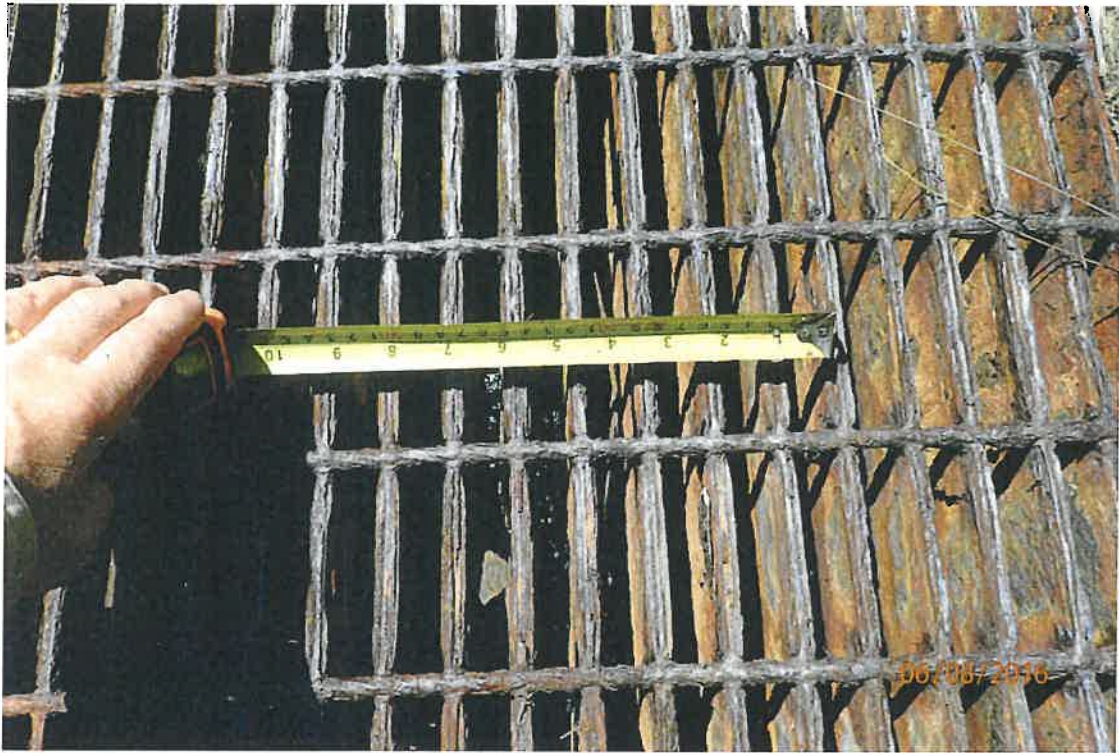
Photo 3: Grating over south upstream flume extension.
