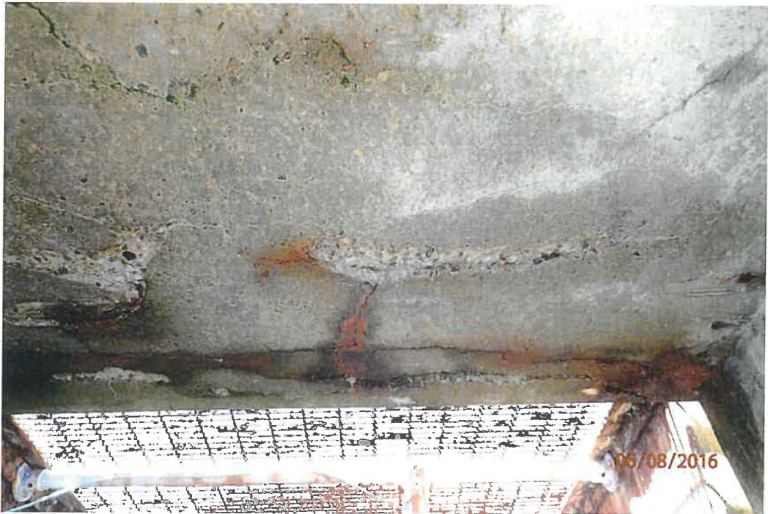
Photo 2: Roof of south upstream flume extension looking west.
