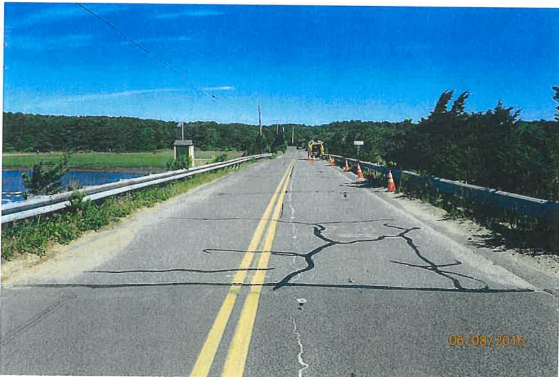
Photo 18: Topside looking north.
