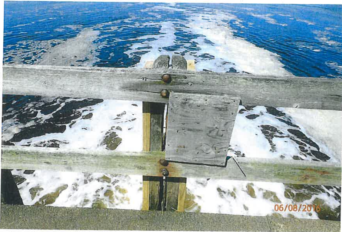
Photo 17: Center post at west has been shored.
