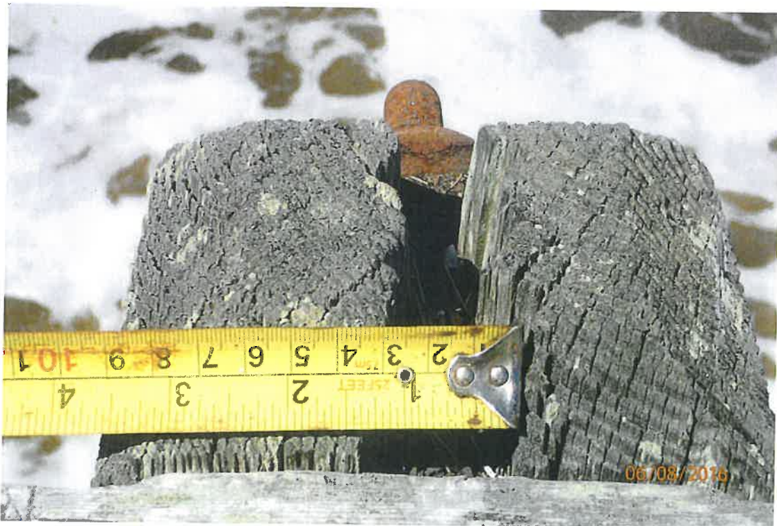
Photo 16: Typical spit in rail post
