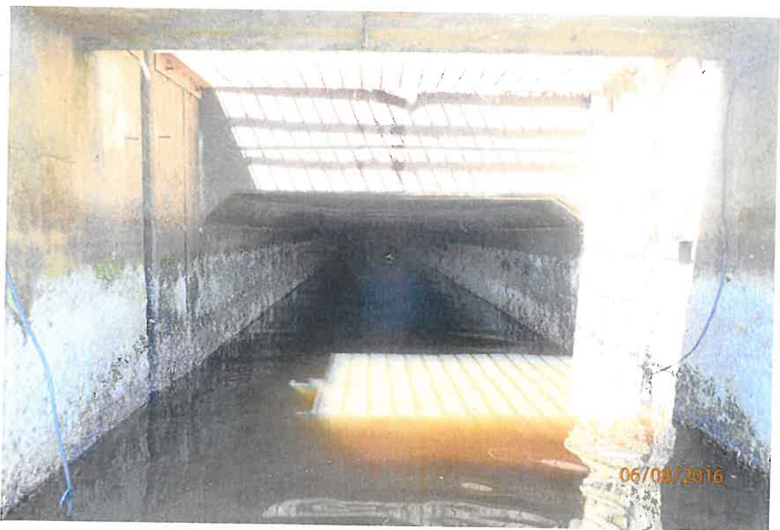
Photo 10: Middle barrel looking west.
