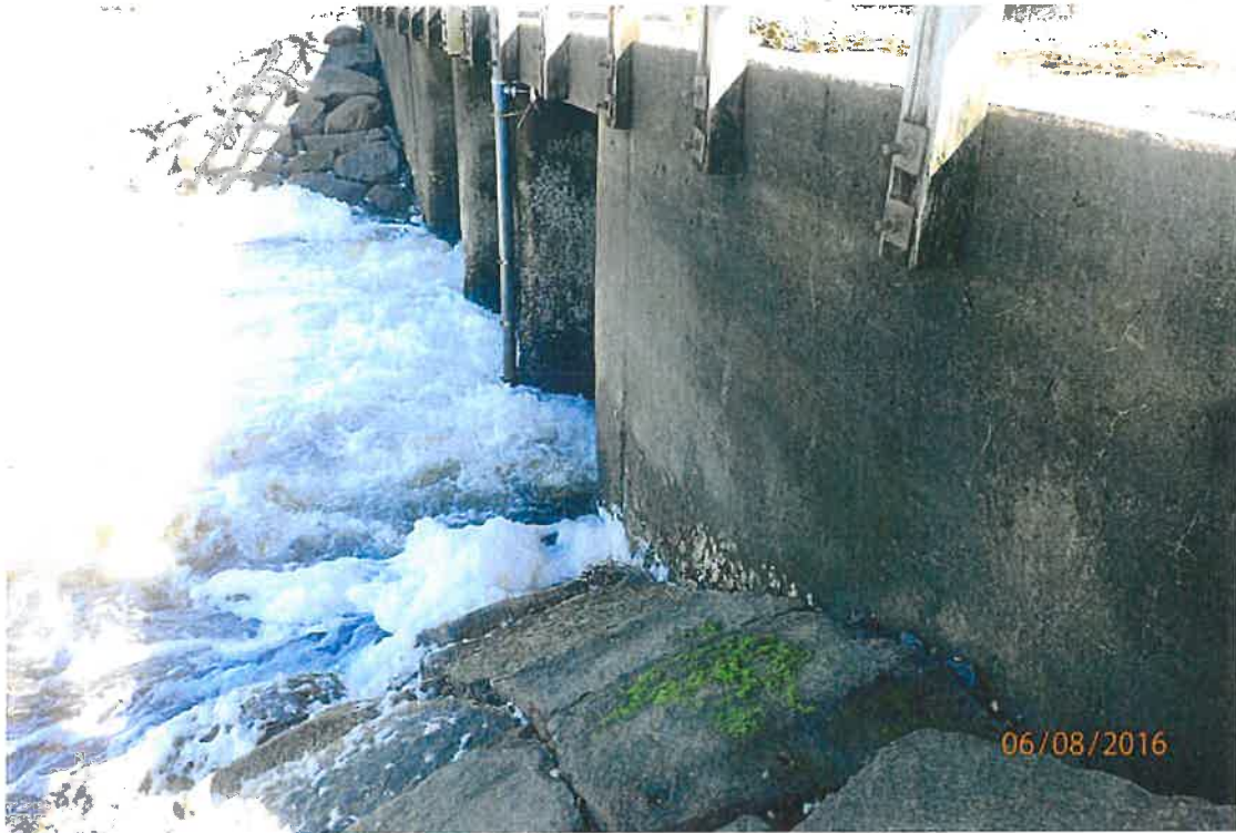
Photo 5: Downstream end, new monitoring pipe installed at end.
