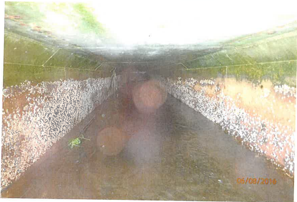
Photo 9: South barrel looking west.
