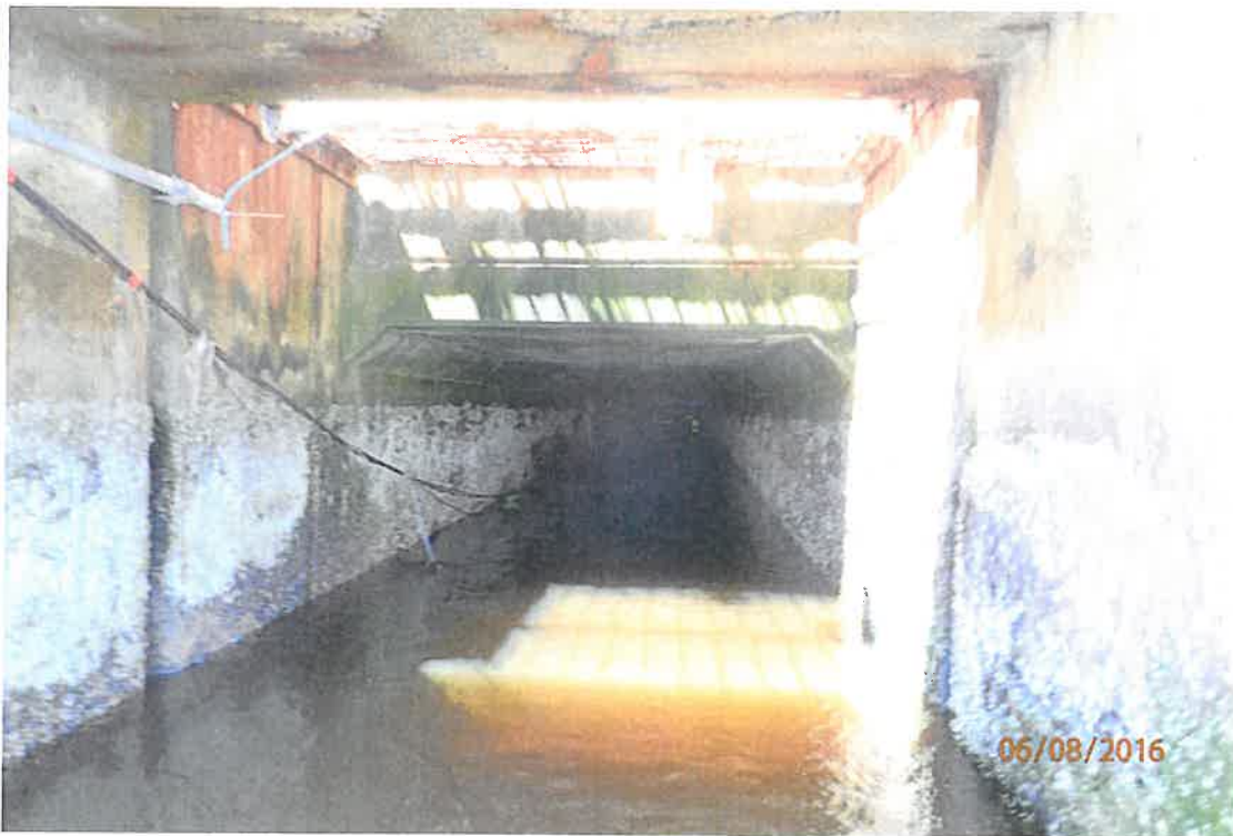
Photo 8: South barrel looking west.
