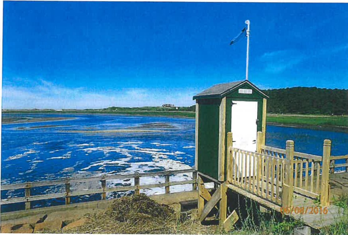
Photo 19: New monitoring building property of the U.S. Government.
