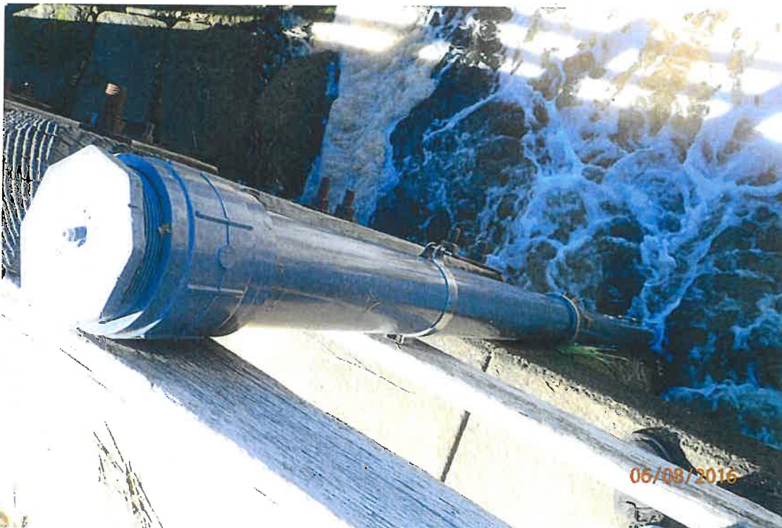
Photo 20: New monitoring duct at the west.
