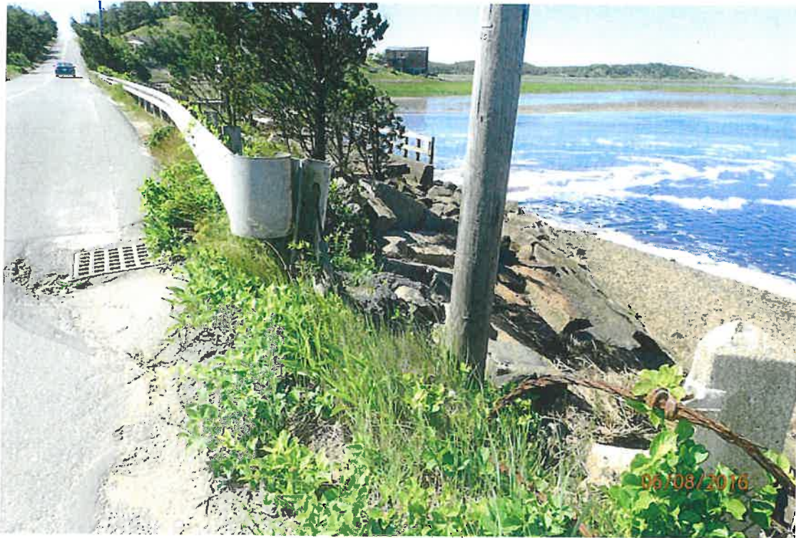
Photo 21: NW gloved end is detached from post.
