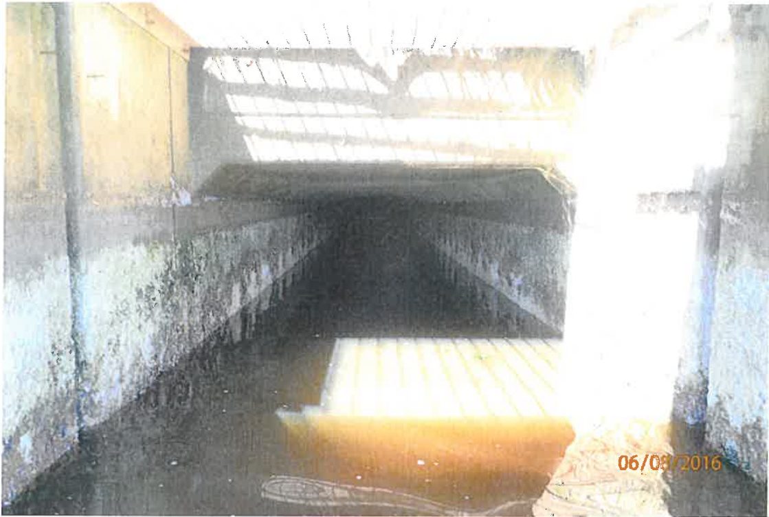
Photo 11: North barrel looking west.
