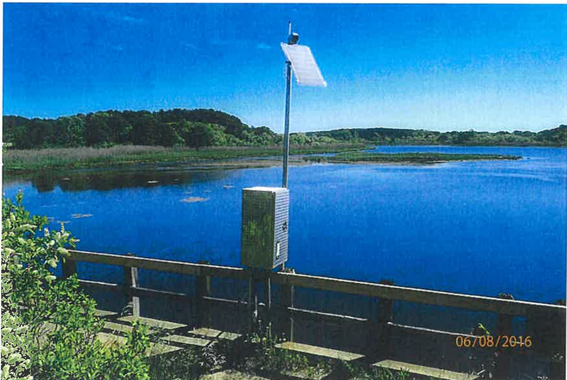
Photo 12: Rail has been repaired at east.
