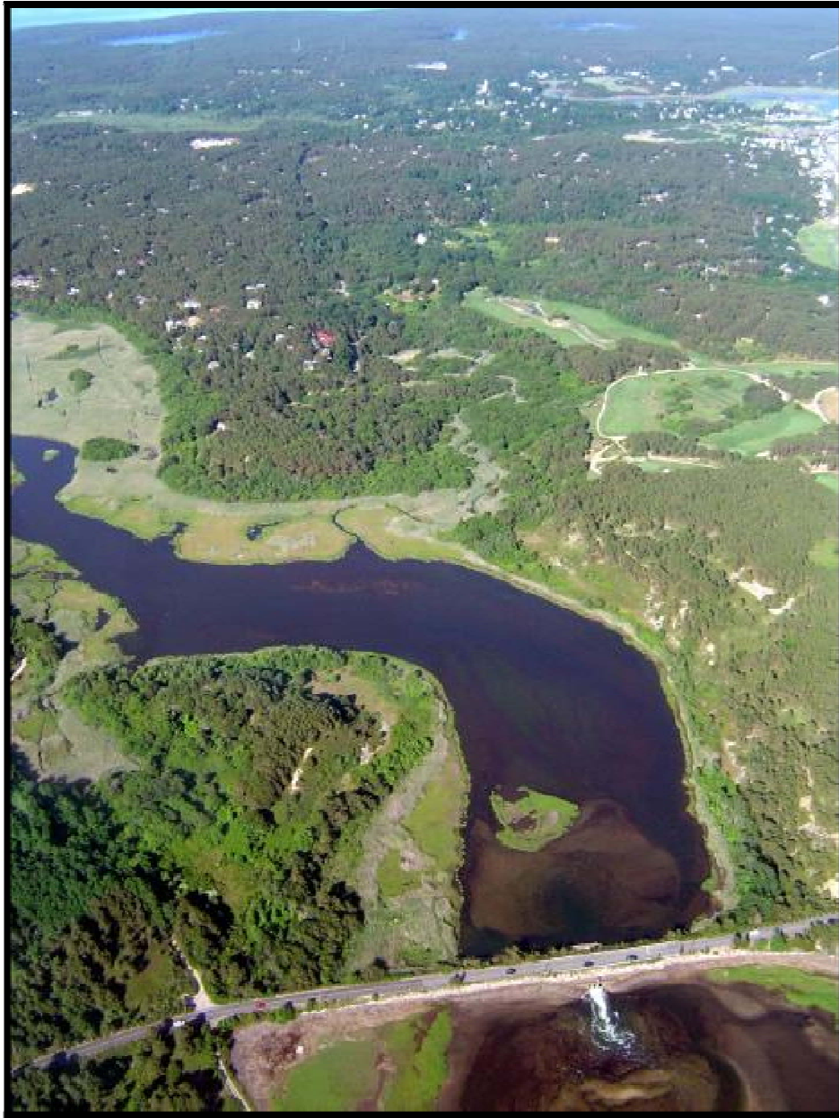
HERRING RIVER RESTORATION PROJECT
