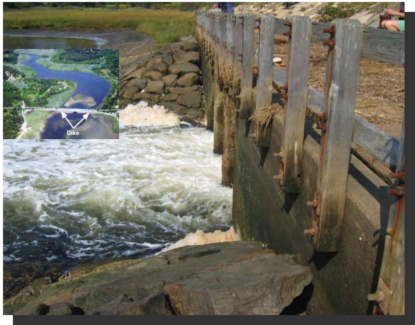
Figure ES-1. Dike structure at the Chequessett Neck Road crossing.
