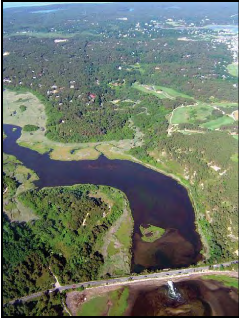
HERRING RIVER RESTORATION PROJECT
