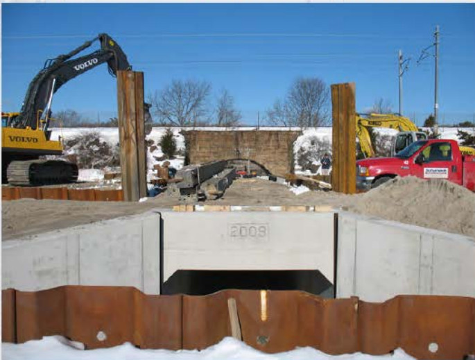
During Construction - Expanded open channel and box culvert under coastal dune
