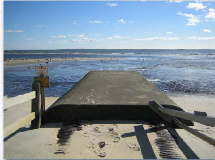
During Construction - Expanded open channel and box culvert under coastal dune
