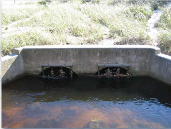
During Construction - Expanded open channel and box culvert under coastal dune
