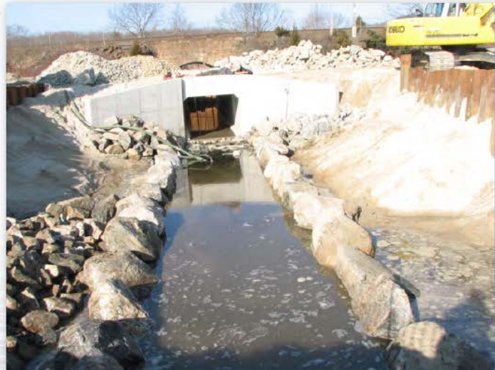
During Construction - Expanded open channel and box culvert under coastal dune
