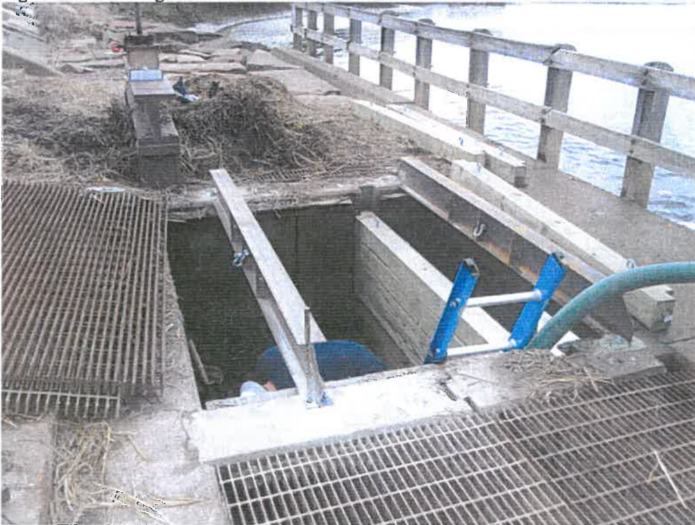
Figure 8: Stop Logs and Reaction Beams Center Barrel Harbor Side Flume
