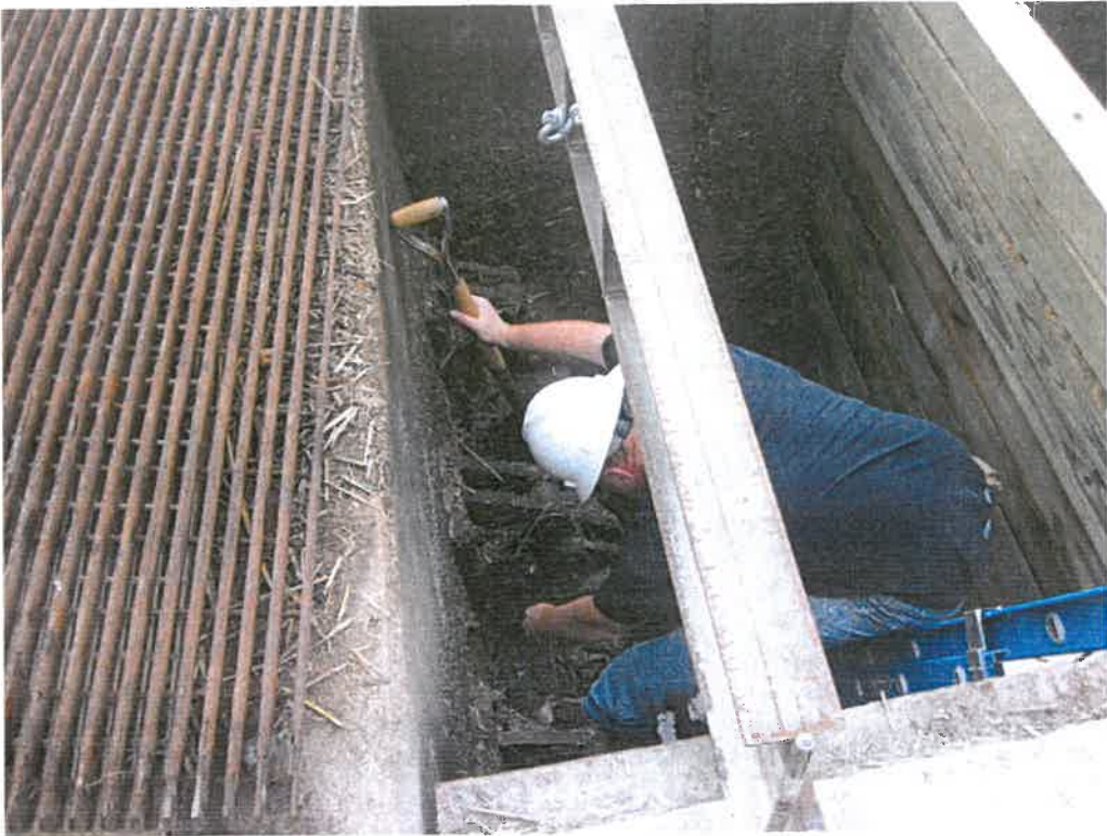
Figure 11: Removing Marine Growth
