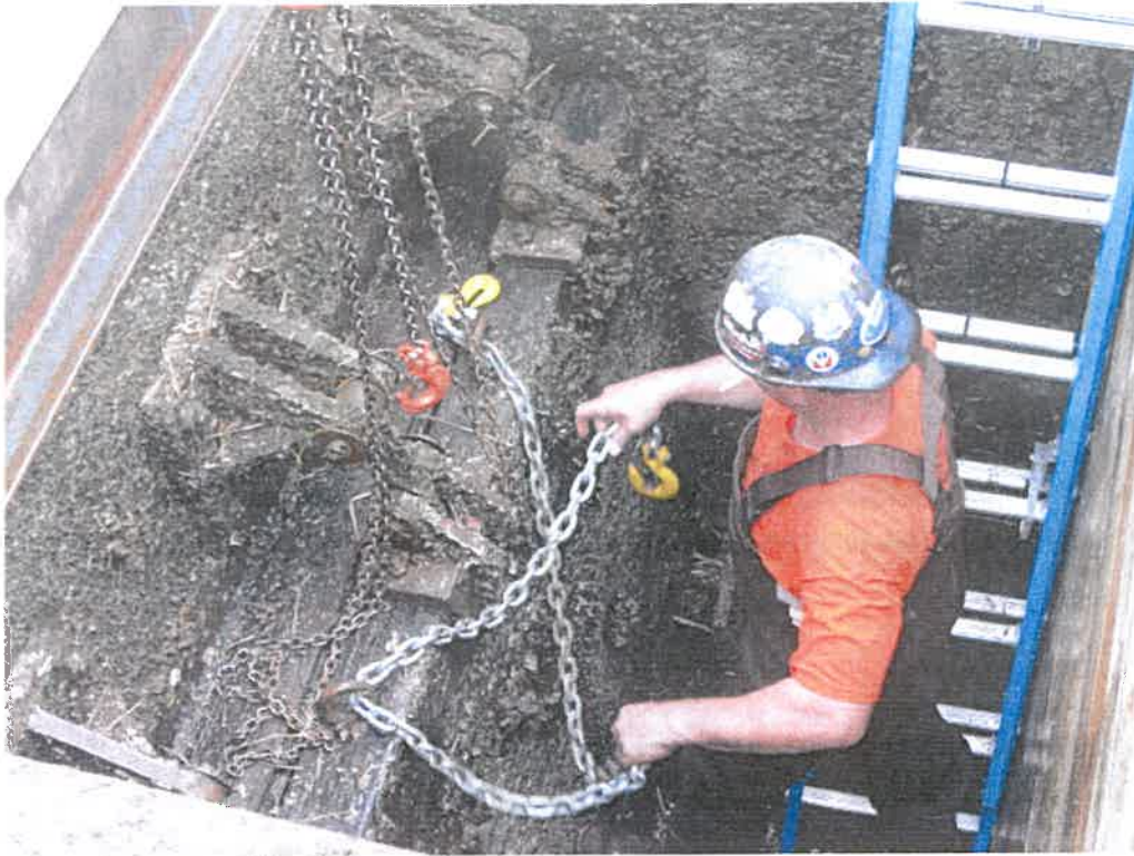
Figure 9: Rigging Tide Gates
