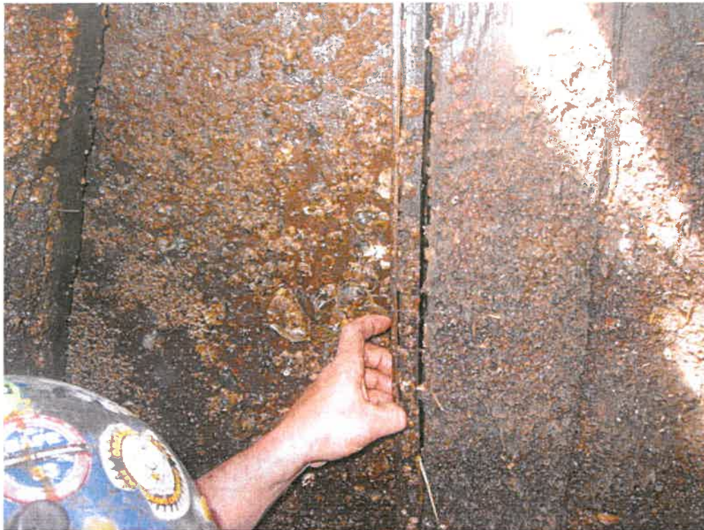
Figure 17: Tee Seal Assembly at Timber Frame North Vertical Center Barrel
