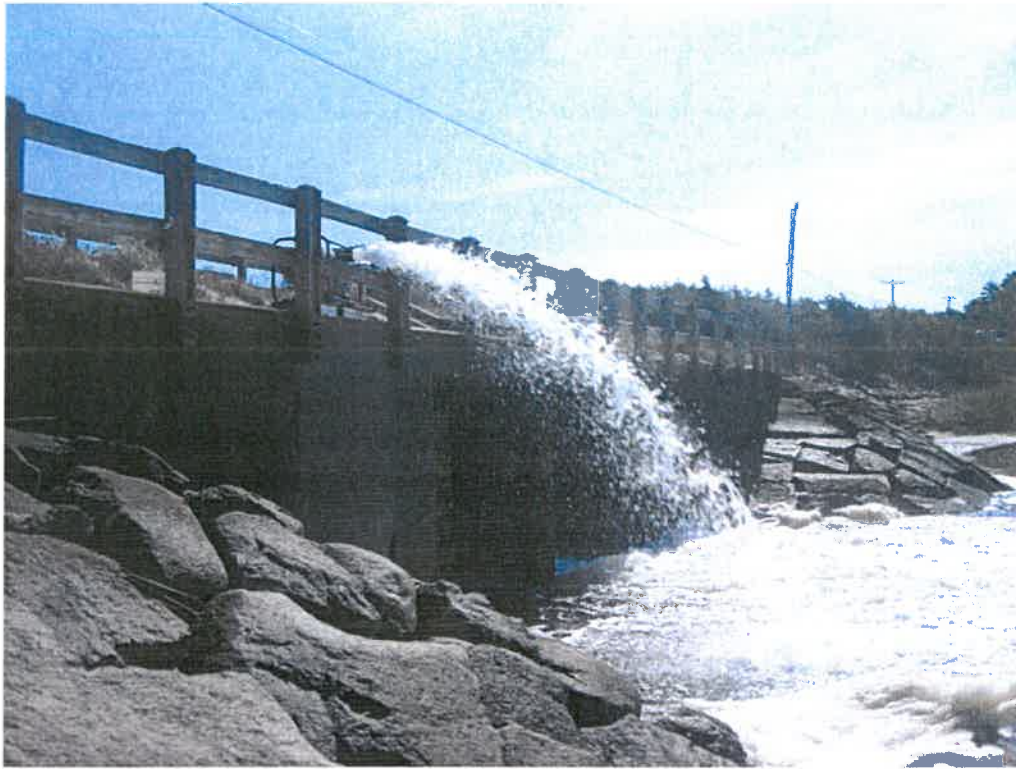
Figure 7 Dewatering North Barrel Harbor Side Flume
